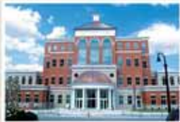
Judicial Center $35 Million project expected completion: 2013
